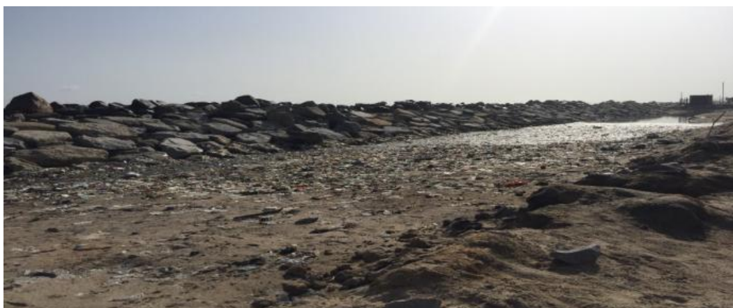
Plate 1.2. Stagnant water (pool of water behind the sea-defense) resulting from water splashed against the sea defense
